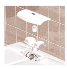
Trap and strainer can be removed to give clear access for rodding
