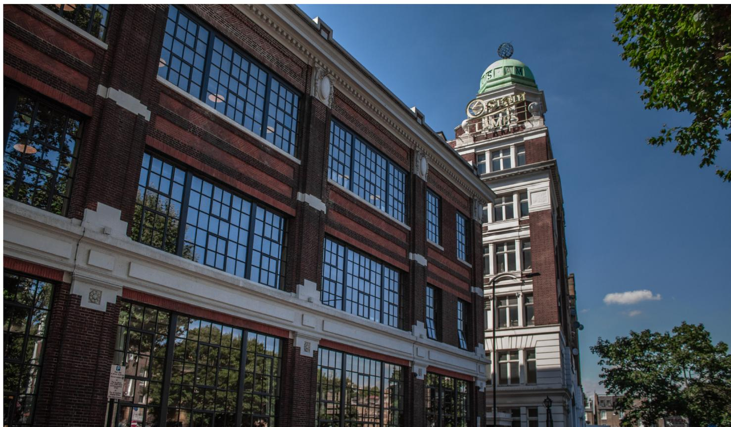
The Berkeley window and door system is an ideal solution for historic projects where minimum sightlines, maximum daylight, and fine detail are desired. Hot rolled profiles feature an external solid steel chamfer that replicates traditional putty glazing in combination with internal beading that offers security and access for re-glazing.
