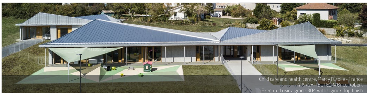
Media library, La Madeleine - France Tank © Julien Lanoo Executed using grade 304L with Uginox Mat finish
