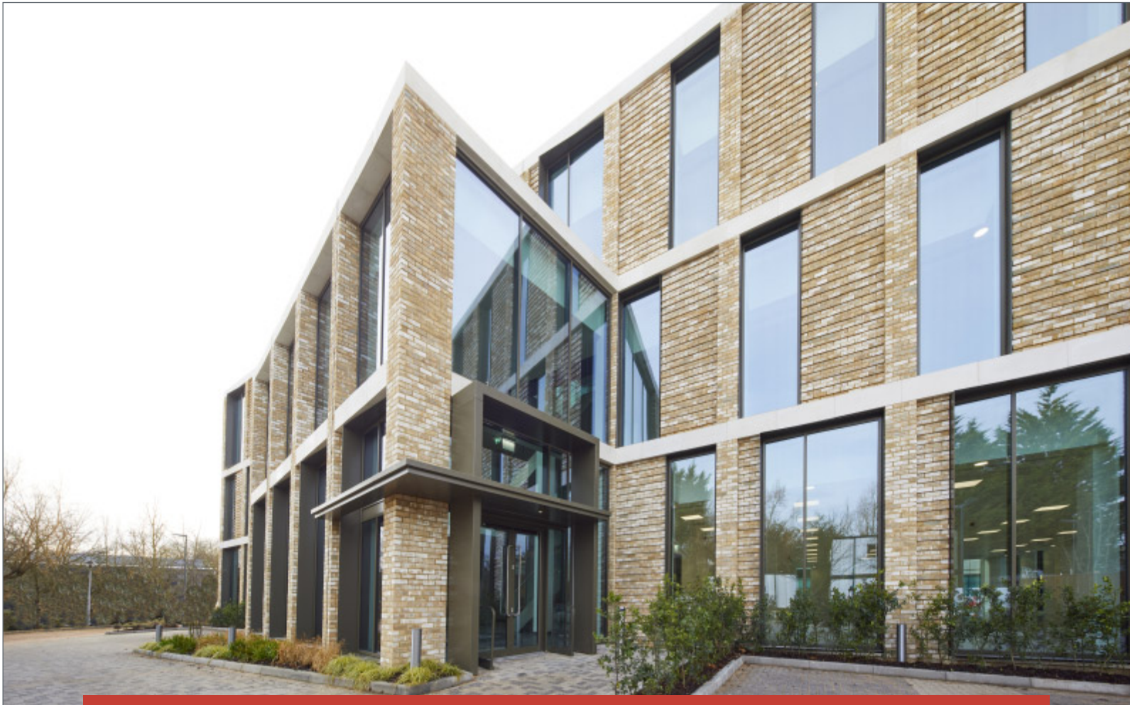
Unit 216, Cambridge Science Park Architect: Broadway Malyan
