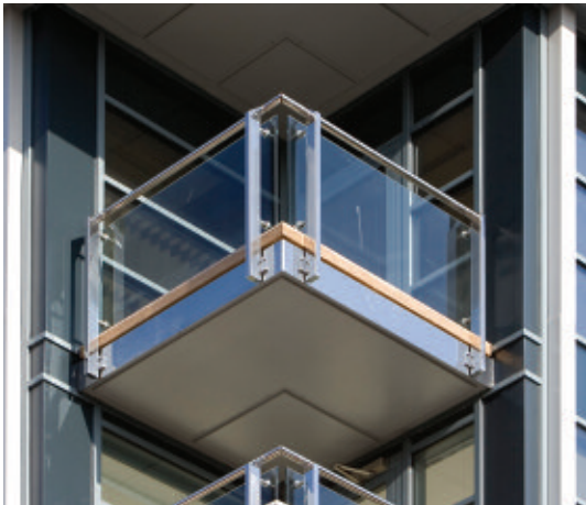
Balcony connection to window system
