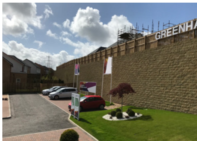
6m retaining wall height on housing development
