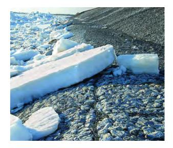
The temperature at which PoliMac® shows brittle behavior is significantly lower than the requirement for PVC, making it more resistant to brittle behaviors at colder temperatures.
