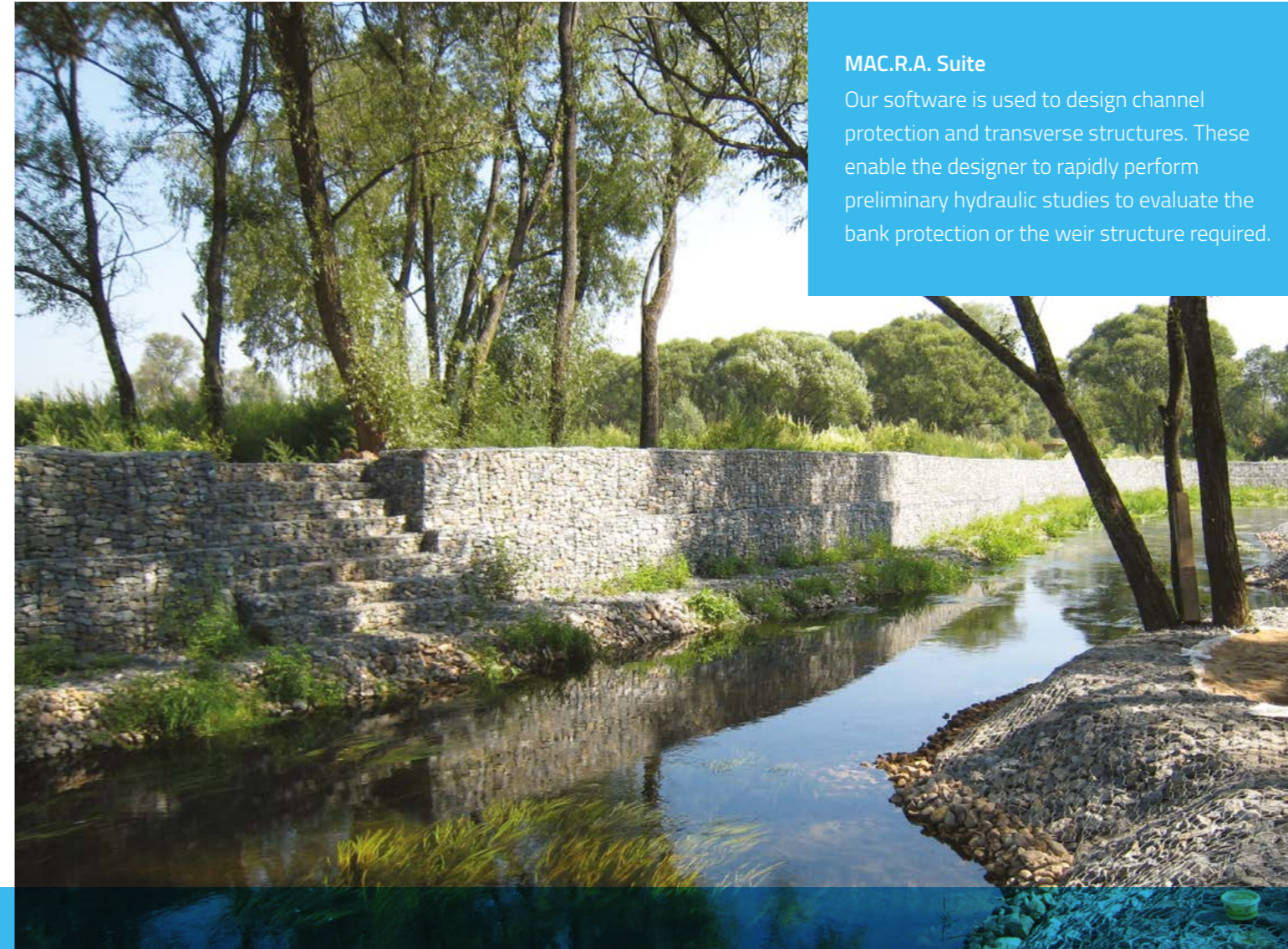
Channelling works containing river in urban area
