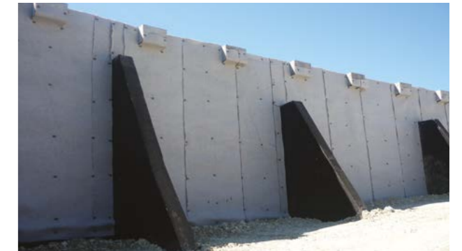
Highway trench drain
