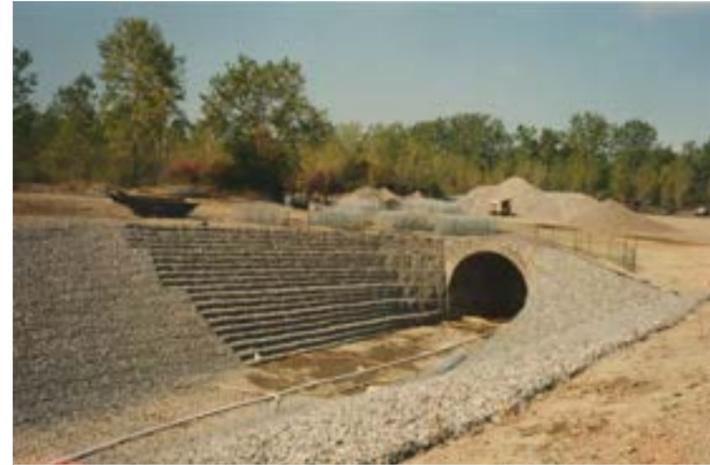
“Gabions and Terramesh® are often used as the culvert headwalls and can be designed to support roadways or other infrastructure above”
