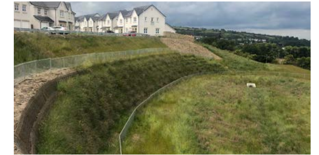
Mineral Terramesh® under construction
