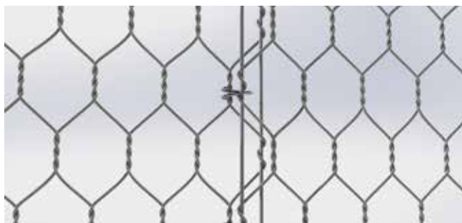
Overlapping of adjacent mesh rolls
