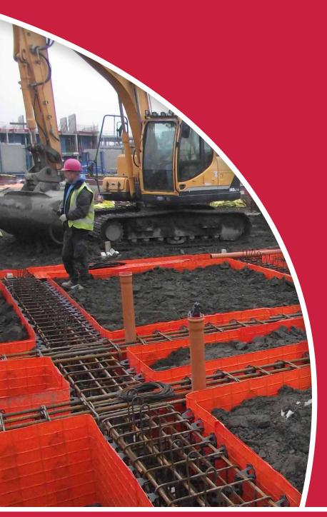
Welded Mesh Formwork System
