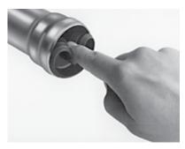
2. Using your index finger to press the seal to one side, push it into the socket chamber.
