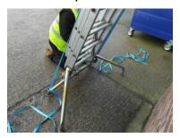
Foot the Ladder or use a suitable Ladder safety device, such as Easi-Dec Ladder spurs before using.
