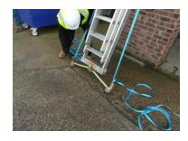
Feed the second tied footing Ladder strap through the second ratchet buckle and then tension both straps making sure the Ladder is vertical when under tension.
