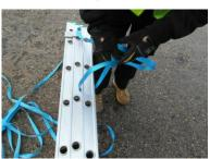
Repeat  $\mbox{\bf STEP~2}$  for the second strap; tie the strap around the third rung and the footing Ladder stile.
