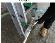
Position the Footing Ladder into the anchor fixing housing.
