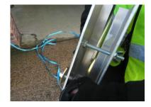
Slacken the bolts on the  $\mbox{\sc Anchor}$  fixing housing.
