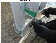
Tighten the bolts from the anchor fixing housing with the wing nuts provided; make sure the Ladder feet are firmly seated.
