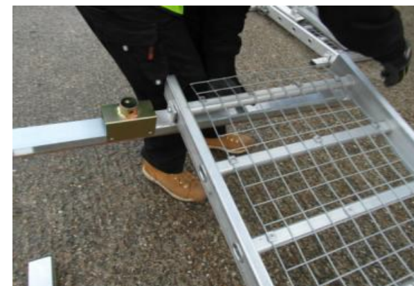
B. Attach the first support batten to the underside of the Board-Walk section using the captivated pins in the holes in the stiles (mesh side is the top)
