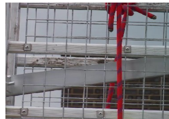
D. Tie a strap or rope to the top rung of the Board-Walk in preparation for lowering it onto the roof
