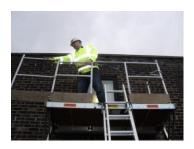
Clip on with a Lanyard and remove the pin and 'R' Clips from the Internal end Guardrails and fold them outwardly, repeat for the second deck. This will provide access for the Catwalk to be positioned.
