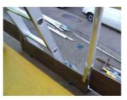
Raise toe-boards across the Ladder access point to complete the assembly  $% \left\{ \mathbf{k}^{\prime}\right\} =\mathbf{k}^{\prime}$
