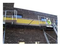
With both operatives clipped on with Lanyards turn the platform on its side and release the towing rope.
