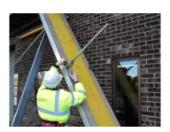
Install the centre posts on the Catwalk and secure with Pin and 'R' Clip. This will allow assembly of the guardrail set prior to access.
