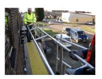
Fit the end uprights and position the front rail over the uprights from the 2m platforms. Make sure each operative is clipped on with a Lanyard. At this stage tighten all grub screws and secure uprights with pin's and 'R' Clip's.
