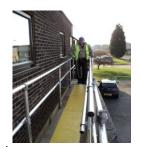
Fit the inner Guardrail the same way as in step 9. Remember to be clipped on with a lanyard at all times when fitting the Guardrails whenever possible
