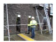
Position the Easi-Decs 4m apart using the Guardrail or staging as a guide. *REMEMBER:* To allow a minimum of 300mm overhang of Catwalk on each Easi-Dec.
