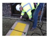
Tie a rope through the Guardrail sockets and secure at the end of the Catwalk.
