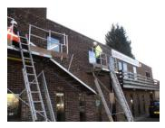
With both operatives clipped on with lanyards the Catwalk can now be raised into position. An operative must hold onto one end and guide while the second operative hoists the opposite end up until the platforms Level at Dec height. The catwalk is then pulled into position with a minimum of 300mm overhang on each platform.
