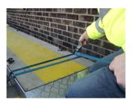
Using the 2 'Ratchet' Straps provided, fix the 'Catwalk' to the Easi-Dec's as shown above. Pass the straps round the 'Horns' of the Easi-Dec frame and catwalk, tightening the buckle in a position where it will not trip the user.
