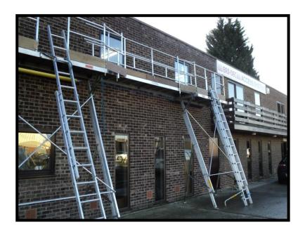
Temporary access device conforming to the test requirements of BS EN 12811 CLASS 2 & EN13774 CLASS C
