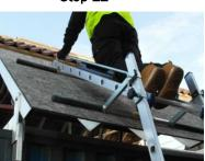
Slide the kneeler to desired position on the roof ladders.
