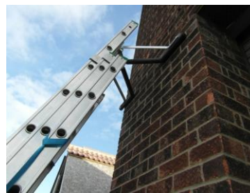
Position the Ladder against the wall or to access corners FIG 1.
