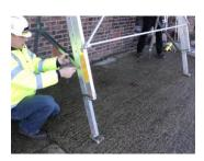
When fitting the Brace the Back Leg Foot should be as close to the wall as possible without fouling on the wall or touching the ground. Fit the Pin and 'R' Clip.
