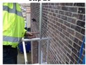
Make sure the support tubes are completely flush with the gate to ensure full connection. **REMEMBER:** Raise the toe-board across the Ladder access point before using the Hoist.
