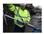
The Hoisting Assembly needs to be secured before lifting, using the supplied Assembly Straps as illustrated. Then tie rope around the top part of the frame ensuring it is properly secure ready for lifting.
