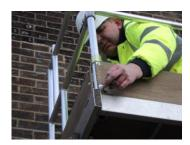
Secure all the uprights in the locating sockets with the Pins and 'R' Clips provided.
