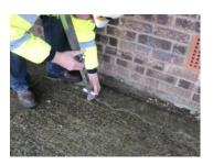
Drop the feet to the ground and take it up to the next hole and secure with the Pin and 'R' Clip. Ideally a finger's clearance under them to ensure the Window-Dec Platform remains in contact with the wall.
