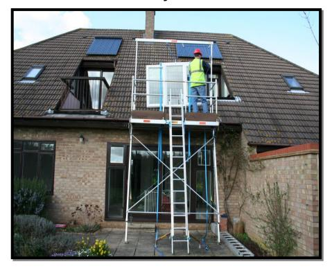
Temporary access device conforming to the test requirements of BS EN 12811 CLASS 2
