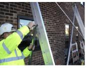
Remove top Pin and fit to the Back Leg at about eye level to the Main Leg.
