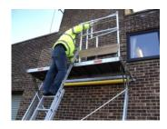
Feed one arm through the top rung of the Ladder and fit the Right Guardrail into the two front sockets and gently ease the back of the Guardrail open. (NOTE: Always Feed one arm through the top rung as this provides a handhold when positioning the Guardrail.
