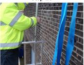
Lift the whole assembly by holding the support tubes and then position these tubes over the Hole in the Guard rail posts. **NOTE:** Two operatives are required to complete the assembly.
