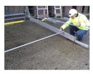
Fit the Horizontal Brace over the retaining studs.
