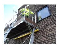
Climb onto the Platform and position the rear Uprights into the rear locating sockets on the platform for both the Left and right handed Guardrail.
