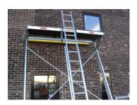
The Ladder is placed against the Platform, extended 1 metre above Platform level between the Ladder Restraints of the Platform and sided to the right to allow enough room to step through on the left hand side.
