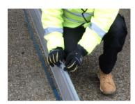
Pull out the clips and release the two Braces from their stowed position.
