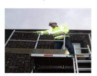
In order to prepare the Mono-Dec Platforms to receive the Catwalks, clip on with a Lanyard and remove the pin and 'R' Clips from the Internal end Guardrails and fold them outwardly. Repeat for the second Platform. This will provide access for the Catwalk to be positioned. Repeat **STEPS 1-20** for the assembly of the second Mono-Dec Platform.
