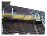
With both operatives clipped on with Lanyards turn the Catwalk on its side and release the towing rope.
