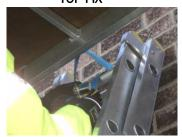
Secure the Mono-Dec Platform to a solid substrate, ensuring the wall tiels securely fixed. Consult a fixing specialist if unsure.
