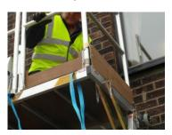
Climb onto the Platform and position the rear Uprights into the rear locating sockets on the platform for both the Left and Right handed Guardrail. Make sure all uprights have been secured with Pins provided.
