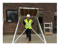
With bent Legs and a straight back, lift the Mono-Dec firstly to waist height, then using your arms to offer it to the wall and roll it up into position.
