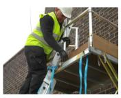
Feed one arm through the top rung of the Ladder and fit the Right Guardrail into the two front sockets and gently ease the back of the Guardrail open. (NOTE: Always Feed one arm through the top rung as this provides a handhold when positioning the Guardrail.
