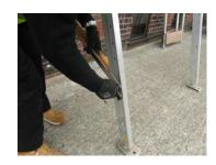
When fitting the Brace the back Leg Foot should be as close to the wall as possible, without fouling the wall or touching the ground. Fit the Pin and 'R' Clip.
