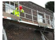
Fit the inner Guardrail the same way as in **STEP 9**. Remember to be clipped on with a lanyard at all times when fitting the Guardrails whenever possible.
