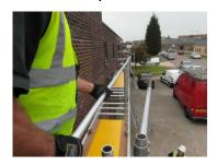
Whilst still clipped on fit the end Uprights and position the front Mid-rail and Top-rail over the Uprights from the 2m Platforms. Tighten all grub screws and secure Uprights with Pin's and 'R' Clip's.
