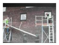
With both operatives clipped on with lanyards the Catwalk can now be raised into position. An operative must hold onto one end and guide while the second operative hoists the opposite end up until the Catwalk is Level at Platform height. The catwalk is then pulled into position with a minimum of 300mm overhang on each platform.
