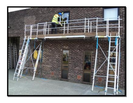
Temporary access device conforming to the test requirements of BS EN 12811 CLASS 2 & EN 13374 CLASS C
