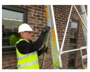
Remove the top Pin and fit the back Leg at about eye level to the Main Leg.
