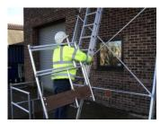
Position the Right Guardrail over your shoulder, when climbing the Ladder, maintain three points of contact. **REMEMBER:** When fitting the Guardrail to the Left hand side of the Platform carry up on the Left shoulder.
