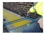
Using the 2 'Ratchet' Straps provided, fix the 'Catwalk' to the Platforms as shown above. Pass the straps round the 'Horns' of the Platforms frame and Catwalk, tightening the buckle in a position where it will not trip the user.
