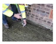
Drop the Feet to the ground and take them up to the next hole and secure with the Pin and 'R' Clip. Ideally a finger's clearance under them will ensure the Mono-Dec Platform remains in contact with the wall.
