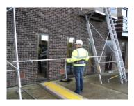
Position the two Mono-Dec Platforms 4m apart using the Guardrail or staging as a guide. **REMEMBER:** To allow a minimum of 300mm overhang of Catwalk on each of the Easi-Dec Platforms.
