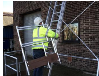
Fig 1 Easi-Dec Ladder spurs.
