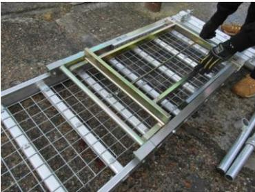
Install the two number trolleys on the separate tracks of Board-Walk. Positioning the rollers on the stiles of the staging and engaging the hooks on a rung.
