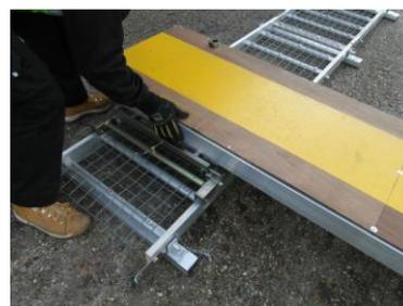
Position the Cat-Walk onto the trolleys.
