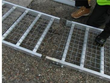
Connecting Additional Board-Walk together, follow **STEP 4 & 5** in these instructions for laying the board walk into position.
