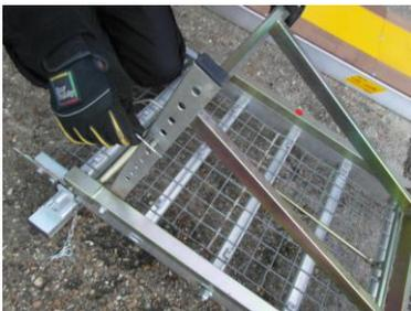
Repeat **STEP 10** for the height adjustment of the trolley on the second roof-Walk in.
