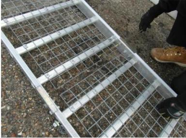
Standing on the first Board-Walk, slide through the Locking pin.
