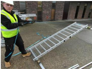
With the strap tied on securely lower the Board-Walk panel onto the roof. You would repeat these steps for additional Board-Walk panels. This picture is for demonstration purposes only.
