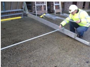
Fit the Horizontal Cross Brace over the retaining studs.
