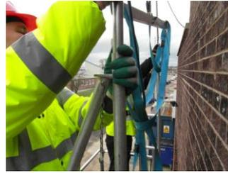
Lift the whole assembly by holding the support tubes and then position these tubes over the Holes in the end support frames.
