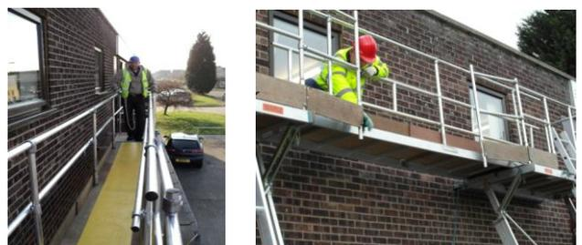
Fit the inner Guardrail the same way as in **STEP 27**. Remember to be clipped on with a lanyard at all times when fitting the Guardrails whenever possible. Secure all Toe Boards to the Uprights.
