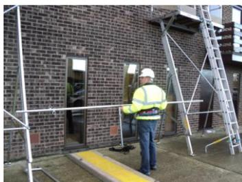
Position the two Platforms 4m apart using the Guardrail or staging as a guide. **REMEMBER:** To allow a minimum of 300mm overhang of Catwalk on each of the two Platforms.
