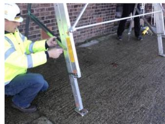
When fitting the Brace, position the Back Leg foot as close to the wall as possible without fouling on the wall or touching the ground. Fit the Pin and 'R' Clip.
