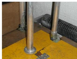
Attach the support frames at both ends to the retaining sockets ensuring the flange is clear of the hatch and flush with the Platform.
