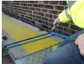
Using the 2 'Ratchet' Straps provided, fix the 'Catwalk' to the Platforms as shown above. Pass the straps round the 'Horns' of the Platforms frame and Catwalk, tightening the buckle in a position where it will not trip the user. **NOTE:** Always ensure the Catwalk is free from obstructing the Solar Platform Hatch.
