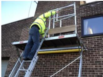
Feed one arm through the top rung of the Ladder this provides a handhold when offering the Guardrail into position. **(NOTE: This is why the Ladder needs to be extended above the platform by 1 metre to provide a handhold)**
