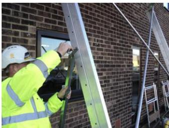
Remove top Pin and fit to the Back Leg at about eye level to the Main Leg.
