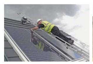
The Solar Ladder offers a safe, practical way of working when installing or maintaining solar panels. The bridging ladder provides 23cm clearance from the roof to the underside of the stile and up to 4.6m free span over the roof. The ladder is simply rolled up the roof on its soft rubber wheels and then flipped 90° into position on the roof. The ladder can also be easily traversed along the ridge with the use of special wheels fitted to the roof hooks.
