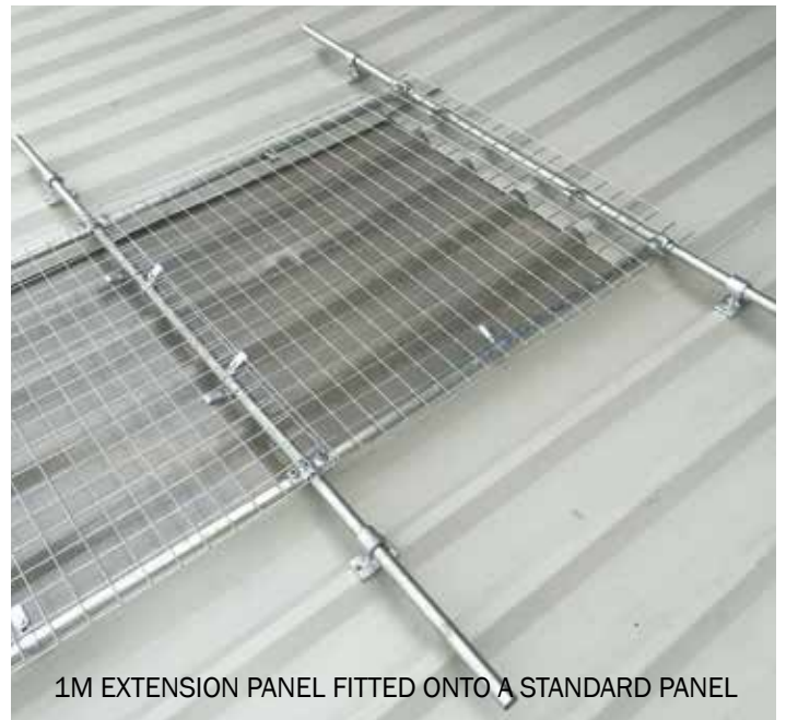
BASE FITTED ONTO ROOF PANEL
