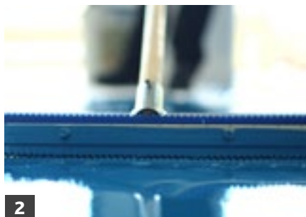
2 Spread with the Resiflow Applicator
