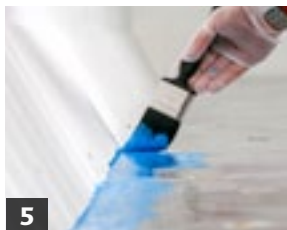
5 Cutting in Do edges first by brush
