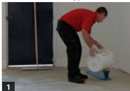
Pour the mixed product on to the substrate
