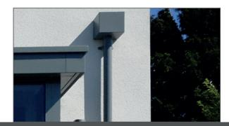
Our hoppers offer a practical solution to increase the capacity of rainwater downpipes and can be designed to match the building aesthetics in both colour and styling. ICB aluminium gutters offer the same high standard, with the benefit of powder coating to any RAL colour. Square or round, they come with a range of gutter brackets to include fascia, rafter-top and rafter-side fixing.
