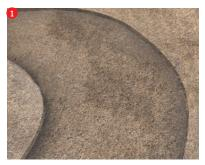
Depending on the soil conditions and intended use of the area to be stabilised, dig out the existing base. Typically, for driveways, 260-360mm.
