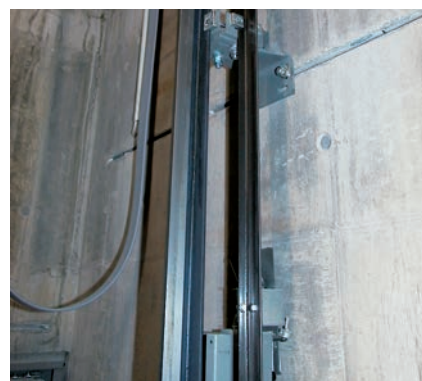
Elevator Guide Rail Connected using Cast-in Channels
