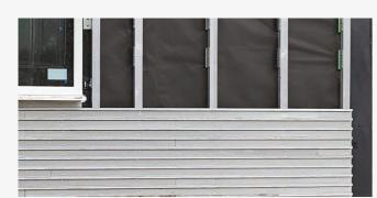
SureBrick can be fixed to many different backing wall types, including SFS, timber frame or concrete.
