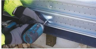
2 Interlocking rails are screwed to the structure, with fixing points at a maximum of 600mm centres.
