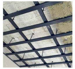
Protektor C3 Coated profiles are designed to meet the requirements for the suspension and support of exterior grade boards in External applications in soffit and wall applications.
