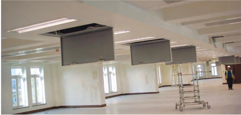
Fire Rated Access Panels provide fire rated protected openings in ceilings and walls for access to building engineering services. Available fire rated up to 2 hours, the doors are finished in powder coated white and can be over painted to blend with the surrounding surface.
