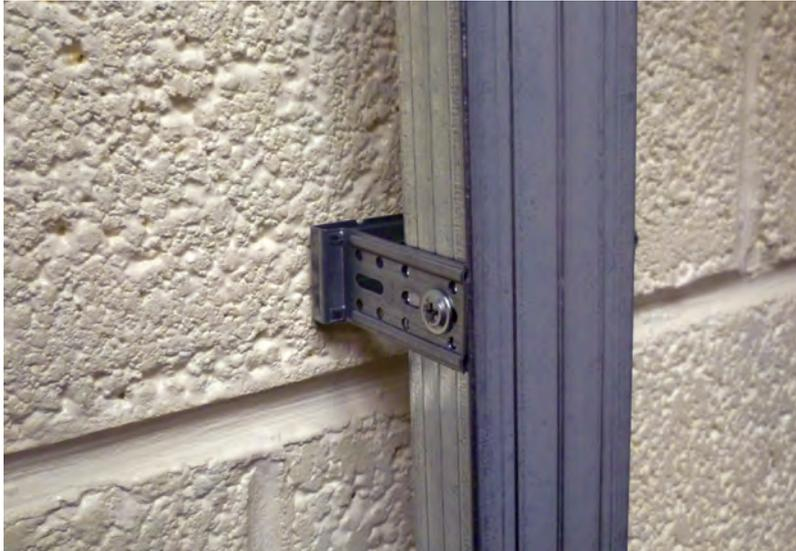
The VCD wall lining system offers a fast, simple to build, method of constructing a steel frame to support a board lining system to solid wall constructions when greater thermal and/or sound requirements are needed.
