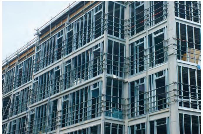
The Protektor SFS system is a widely recognised and proven method of creating external and internal stud frames across a wide and diverse range of construction projects.
