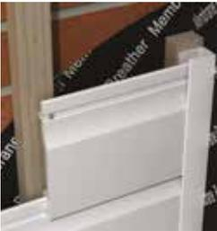
Two-part edge trim to finish a cladding cut back on its length to accept the expansion of the board
