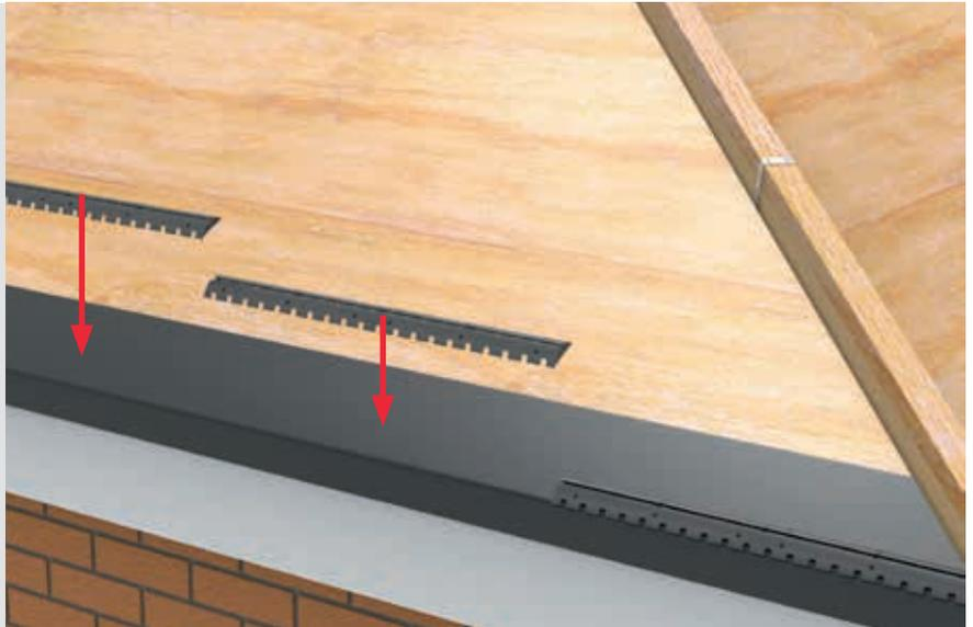
Starting at the right hand edge of each roof face, run through the full roof width with Eave Bar/Starter Rails, ENVEB.
