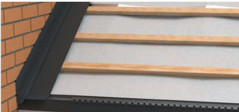
When the abutment soaker is secured, fit the final starter rail as shown, screwing through the abutment soaker.
