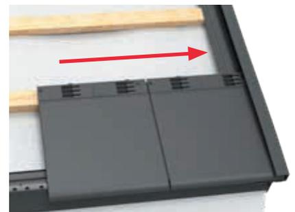
The spacing between tiles can be adjusted to allow for course length (see next stage), but ensure that the minimum spacing is 5mm, and that the fixing hole (A) comes over slot (B) when the tiles are joined.
