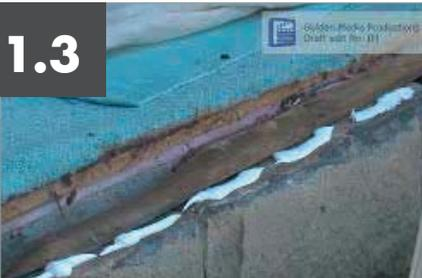
Apply a generous bead of silicone across the bottom of the aperture to sit the base cill on and fix the cill to the aperture ensuring that it is level.
