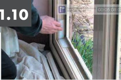
Fit the glass and pack appropriately. All sashes must be toed and heeled to ensure an equal and parallel sight line between the head of the sashes and the outerframe. When the glass is fully packed out, re-bead placing the beads in their original locations.
