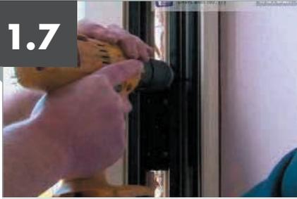
Fixing distances: corner fixings shall be a minimum of 150mm and a maximum of 250mm from the corner. Intermediate fixings shall be at centres no greater than 600mm.
