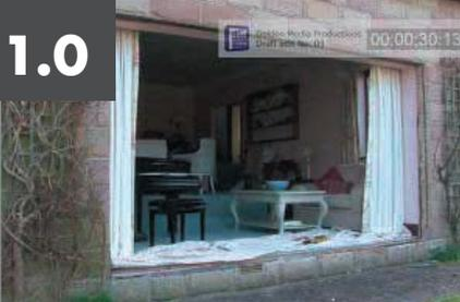
Before installing the Aspect door, the structural opening should be cleared of all dust and debris, and a check made to ensure the D.P.C is in position and is undamaged.
