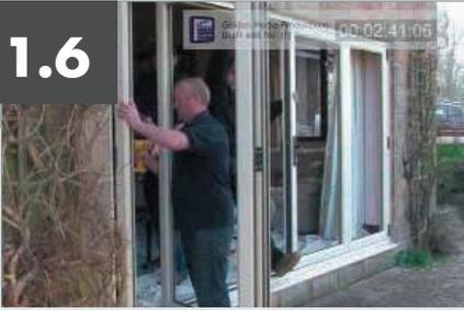
Once in the correct position and the door is plumb and square without twist, you can begin fixing the door into the opening, using appropriate fixings (not supplied). When fixing down to the cill, ensure that screws are sealed to prevent water ingress. Also seal across the cill below the door jambs to prevent water tracking across the cill.
