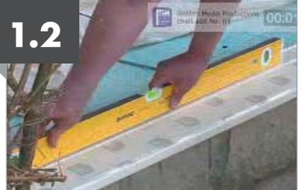
Offer the base cill into the opening, check the cill is level across its overall length (maximum deviation is 3mm).
