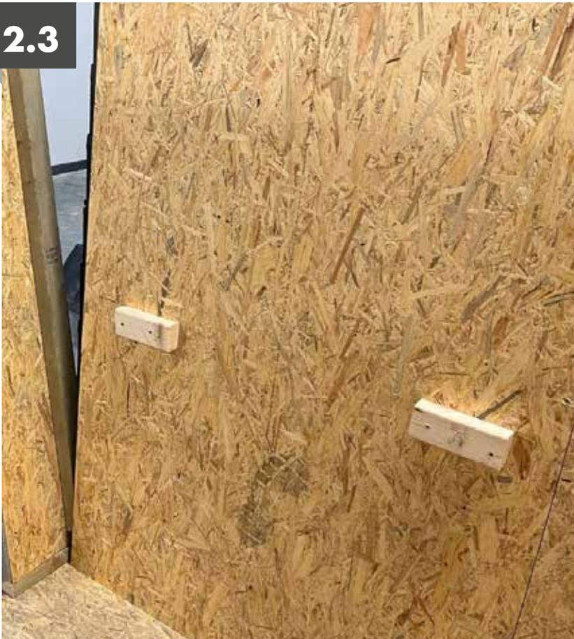
Lift the rear corner panel into place and slot it into the side panel.
