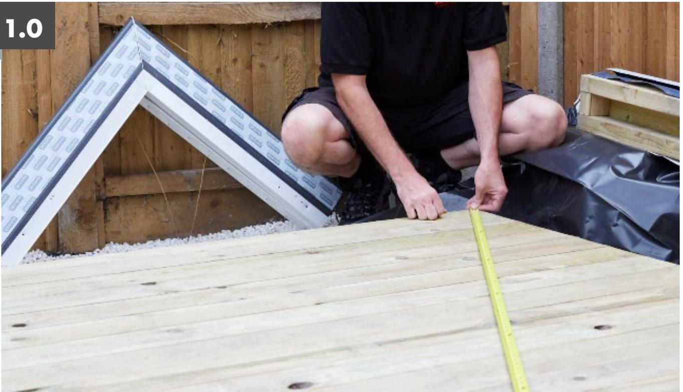
Ensure the base is clean and level. Take care to sweep away any loose gravel etc as this can prevent the floor panels slotting together.
