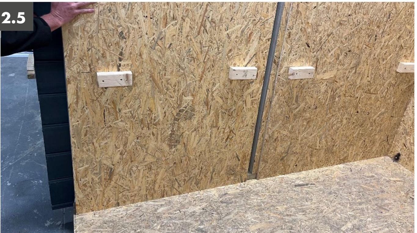
Continue to fit the remainder of the wall panels. The side and back panels slide together as shown below and are also secured either side where they join both vertically and along the base where they meet the base plate.
