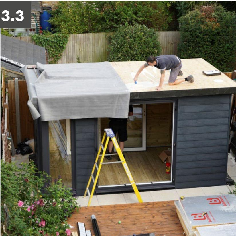
Lay the rubber over the adhesive ensuring no air bubbles (use a lean sweeping brush if required to remove them).
