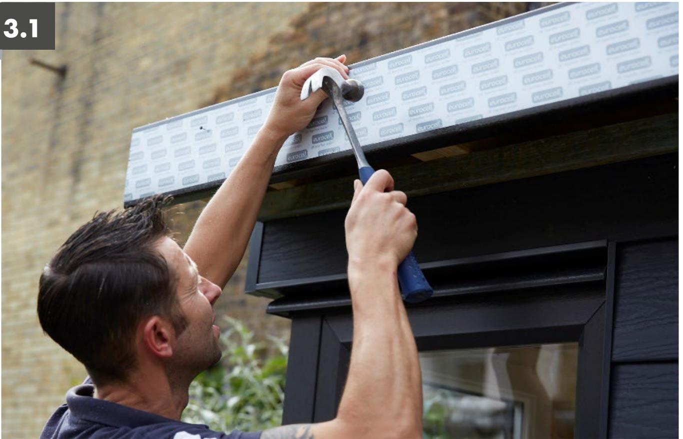
Fit the larger fascia boards to the roof as shown above using the poly pins provided. The top of the fascia board should align with the top of the roof at this stage.
