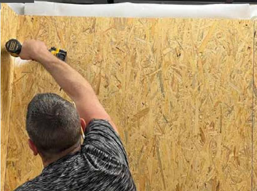
Where the panels meet screw from the inside to secure them together both vertically and along the base plate.
