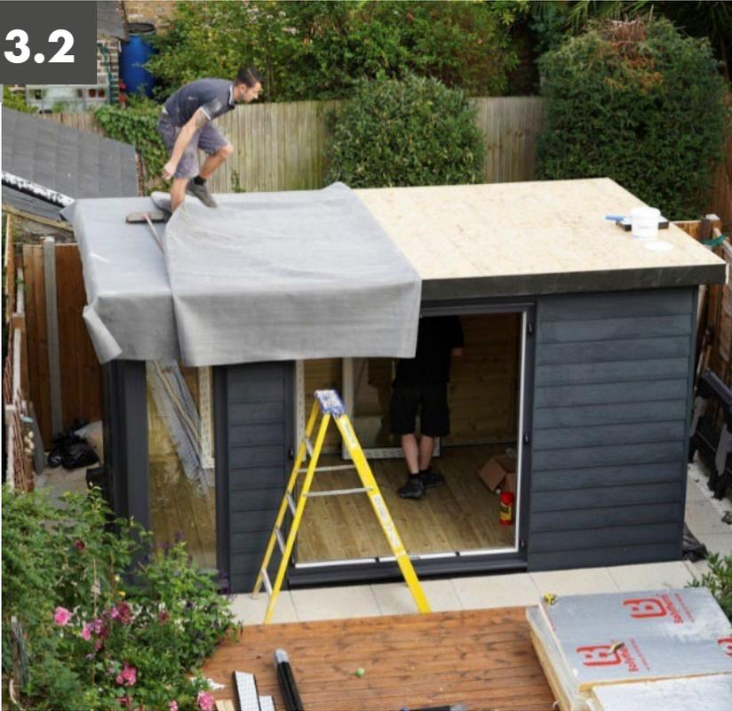
Very carefully lift the rubber onto the roof and spread it out with an even overhang.
