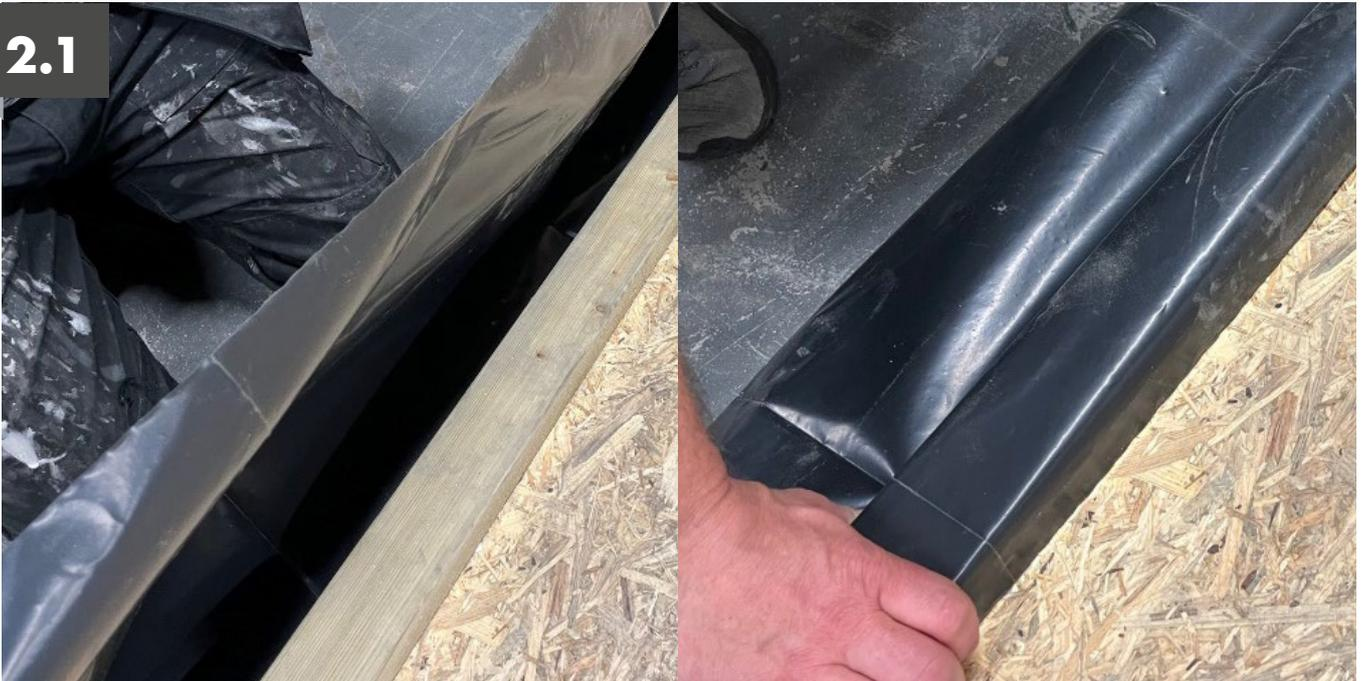
Fold the Damp Proof Membrane over onto the floor (this can be trimmed back later).
