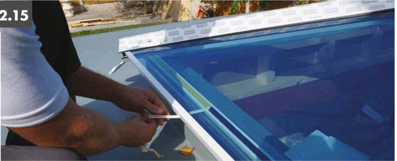
Fit the rafter and hip top caps using a nylon mallet, then ensuring the glass is positioned correctly, peel the remaining eaves beam seal tape film away and press glazing down to ensure contact with eaves tape.
