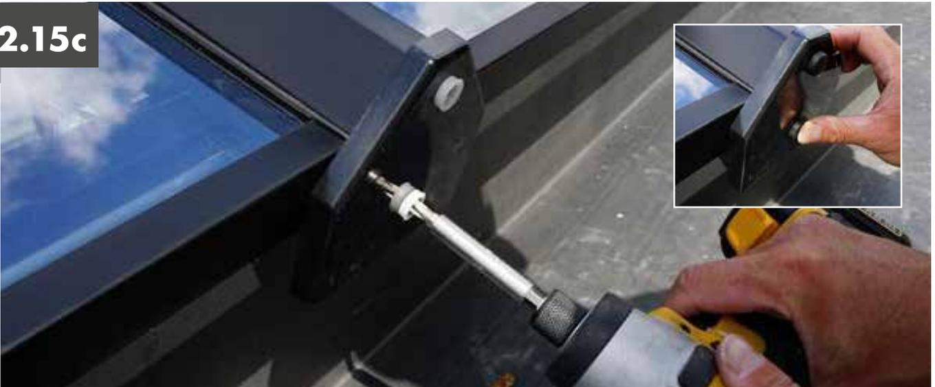
Protective film can now be peeled off and then glazing stops plus end plus end caps fully tightened and secure.
