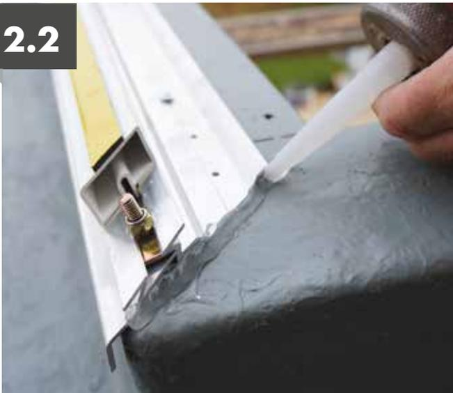
Run a bead of silicone sealant along the mitred edge of the ring beam to seal the corner joint, when the next ring beam is offered up.
