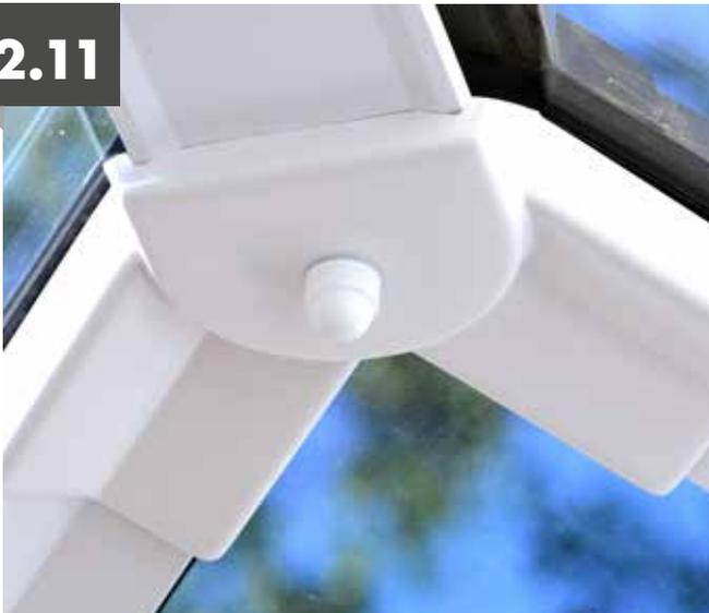
Position the spider bottom cap and fix using the decorative boss onto nylon threaded bar. Note the nylon bar may require trimming down in length.
