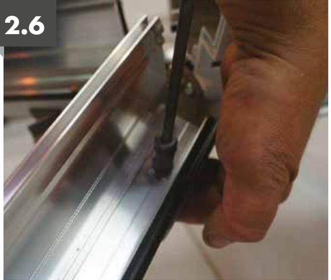
Using 2 x CRS8624S single studs, secure each hip to the spider casting. The body of the stud should locate between the retaining ribs on the lower casting face to stop the stud from spinning.
