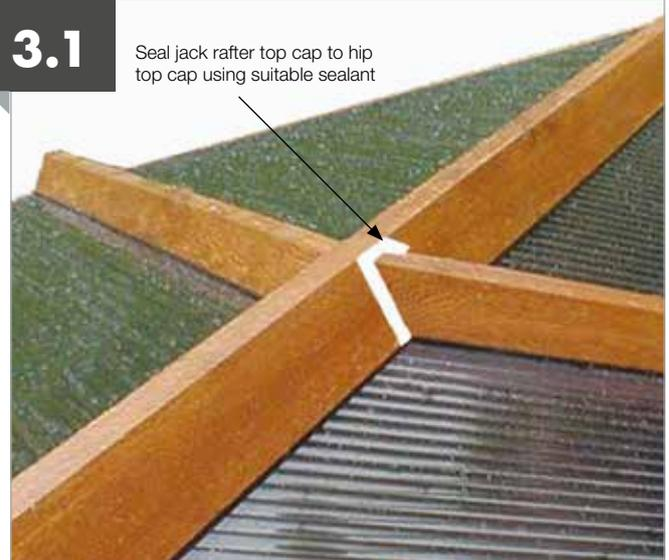
Seal jack rafter top cap to hip top cap using suitable sealant
