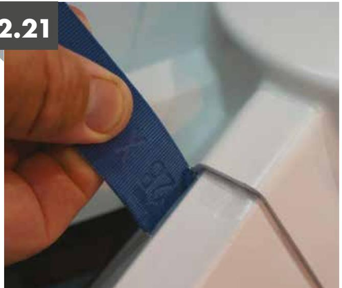
Ensure the capping is seated down correctly and remove any excess sealant from all edges.
