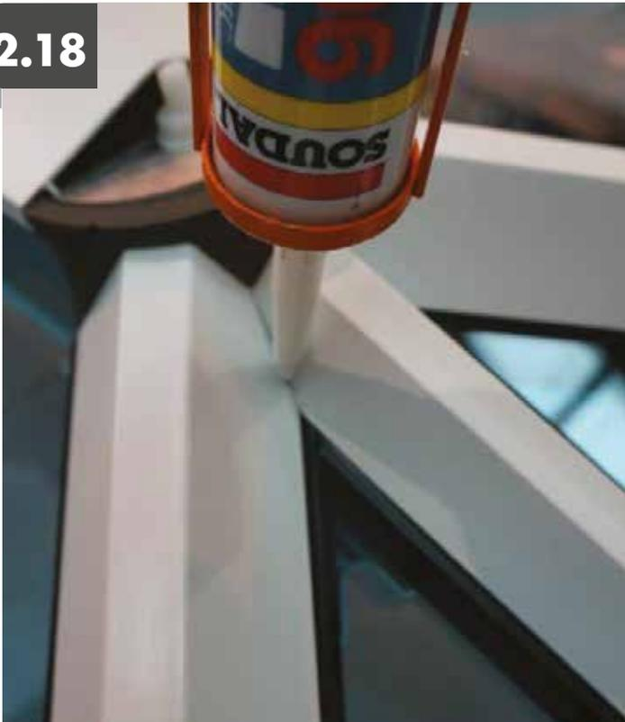
Seal the rafter top cap to hip top cap from the gasket intersection to foam bung.
