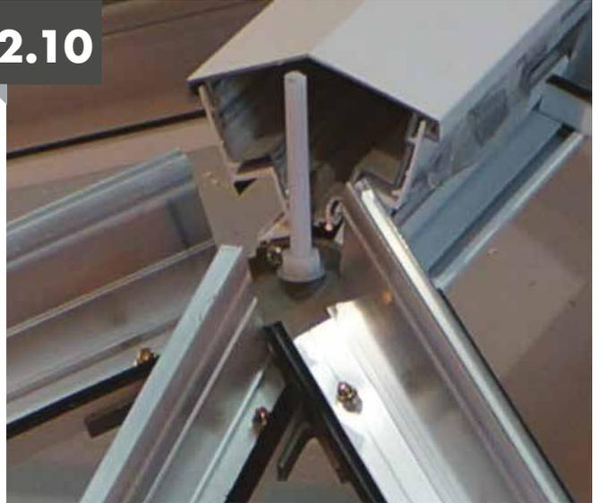
Locate the nylon bar through the spider and lock off using nuts and washers either side of the spider. The nylon bar should sit 5mm below the crest of the ridge profile.
