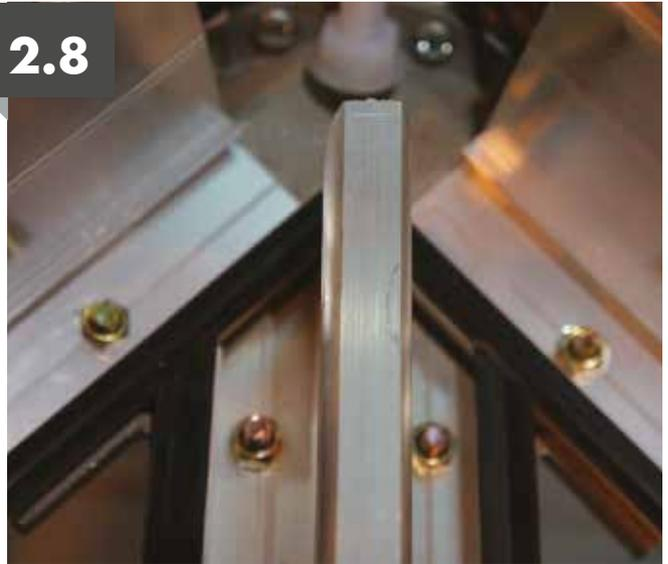
Fasten the central rafters to the spider using 1 x CRS8625S double stud and nuts. If jack rafters are present, please refer to Section 3: Installing Jack Rafters on page 13.
