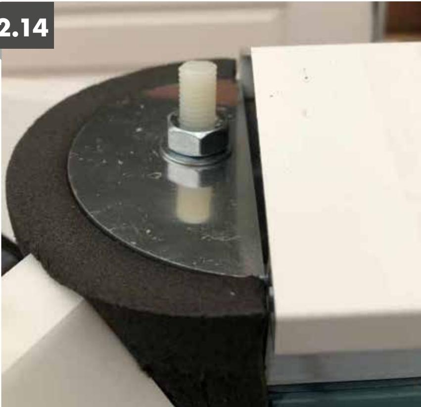
Fit the foam bung and clamp plate and tighten M10 nut until the foam is firmly pressed down onto glazing.
