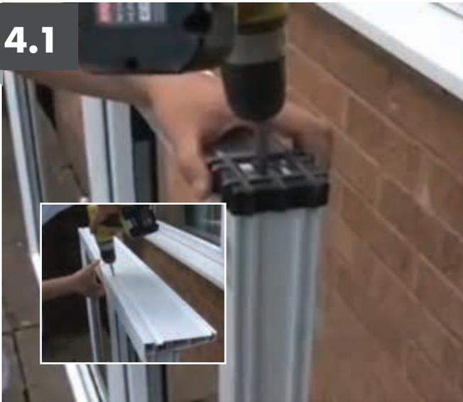
Remove any packaging from the new frame. Apply a bead of silicone along the length of the frame where it will meet the cill.
