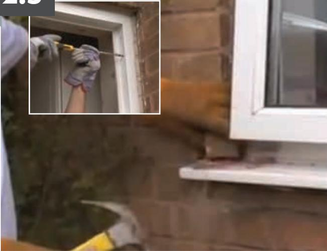
Remove any old fixings and break the external silicone seal with a blade. Also remove the external brick corners to release the old frame.
