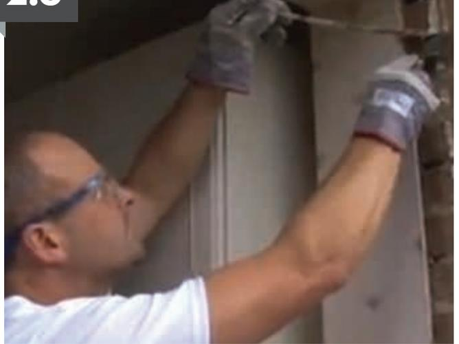
After the removal of the frame, remove all sealant and debris from the brickwork.
