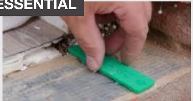
Always put a **4mm packer** under the hinge side leg. If the lock side needs lifting or dropping to square up the head you now have some room for that adjustment. Also seal with silicone between the threshold and cill to stop water ingress.
