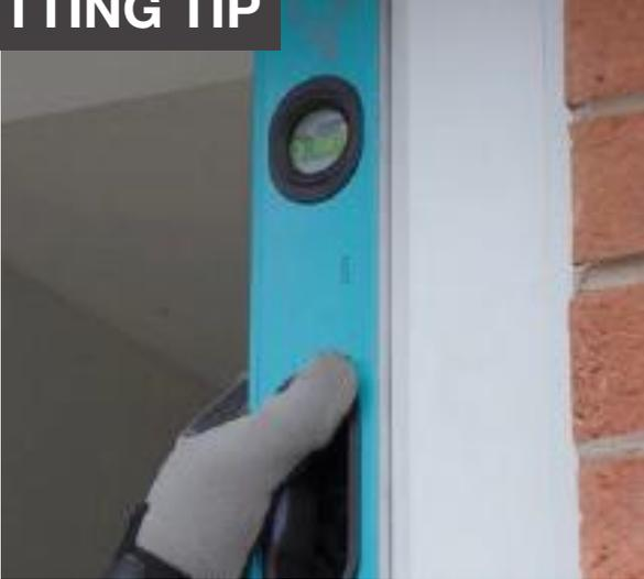
Remove the rubber from your level and get it right into the top when squaring up, you may find the frame is bending inwards in the top corner. This bending in of the frame causes issues with the way the sash hangs square.
