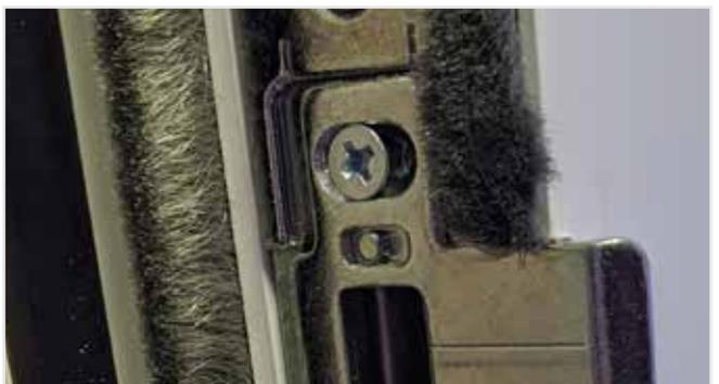
The top and bottom keeps can now be adjusted in the same way but the hooks should hit the plates so that they just pull the sash into the gasket slightly.
