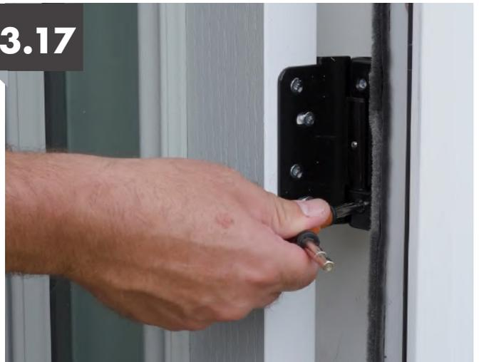
If hinge adjustment is required, the hinge can be moved left to right using the side hinge. Quarter of a turn should be sufficient, ensure that the top and bottom are both adjusted inline with each other on each hinge
