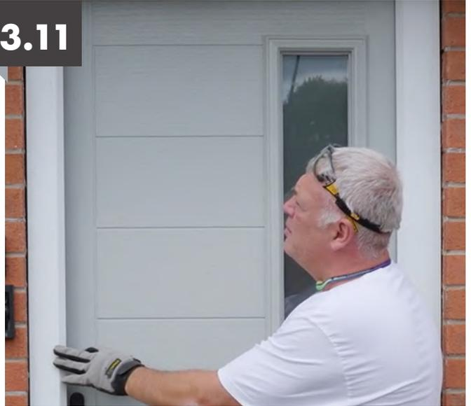
Bring the door slab to the frame checking that it touches top and bottom before the centre fixing is installed
