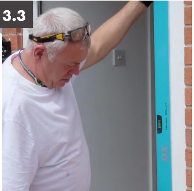
Using an 1800mm level, check the frame is plum
