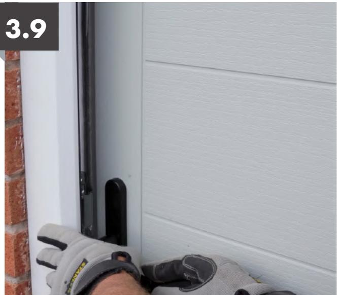
Bring the door slab to the frame checking that it touches top and bottom before the bottom fixing is installed
