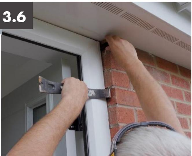
Using a crowbar to move the frame over, insert a 4mm/5mm packer at the top of the frame. This is to stop the frame from pulling over when the next phase of fixings are installed. This ensures an equal air gap between the two brush piles.
