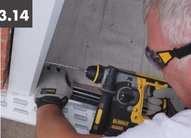
Install the remaining fixings, on both the hinge and keep side of the door, there should be 6 fixings in total on either side, with a fixing above and below each hinge and keep. Ensure a 5mm pilot hole is drilled in the frame prior to fixing to the brickwork.
