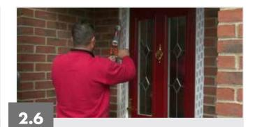
Expanding foam should now be applied between the frame and brickwork ensuring only enough is used to avoid distorting the frame when it expands. Once the foam has dried it can be cut away and perimeter sealing can be carried out. Ensure the frame is free from dust and debris before applying silicone. Do not seal across the front of the aluminium threshold as the drain holes are concealed behind the front ramp.
