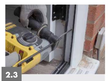
Second fix should be placed underneath the bottom hinge making sure the hinge side leg is plum and level using packers where required to prevent any twisting.
