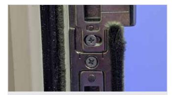
Loosen the adjuster plate by turning the screws anti clockwise one/two turns maximum. Move the latch plate in 1 to 2mm and re tighten screws, close the door using one finger against the door leaf, it should latch easily without any 'rattle'. If it will not close, back the plate off slightly, if it 'rattles' move plate further in and carry out check again.
