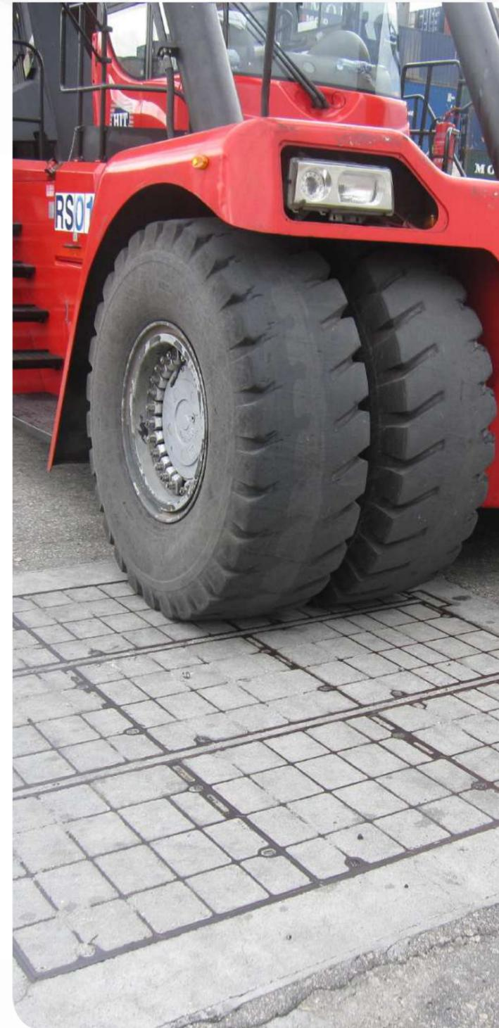
Constant movement of containers and heavy loads in and around ports and storage facilities puts a tremendous load on surface components, such as access covers. Anything that doesn't fit exactly will soon develop rock, which will eventually lead to failure.
