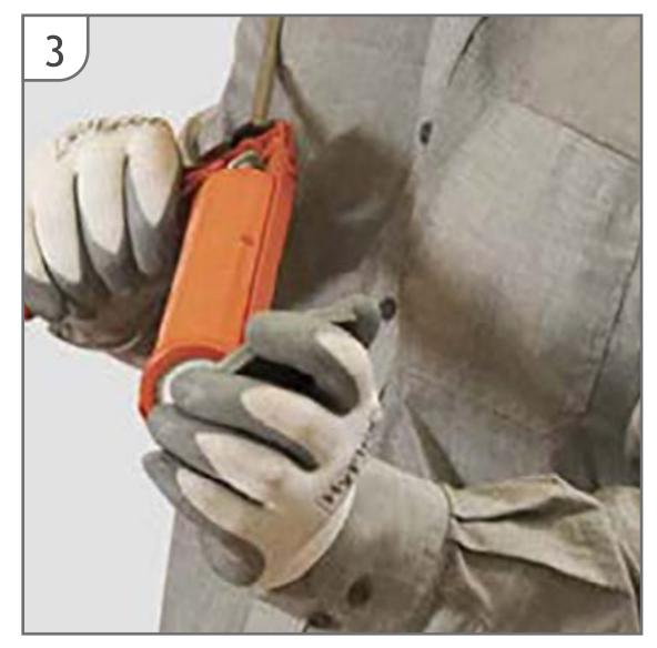
Use the Quartz Zinc adhesive to seal and fix the stop end. To avoid cuts from edges, always wear gloves when handling zinc components.
