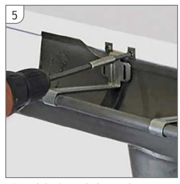
Do not fix brackets to the fascia until gutter is joined to the next length.
