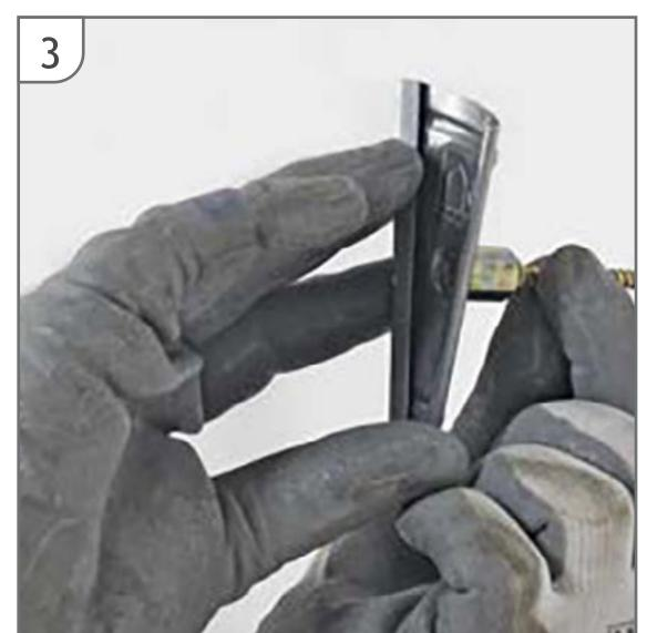
At downpipe joints, mark positions for the v-locks at every 2 metres (maximum). Then firmly screw-fix the v-lock to the wall.
