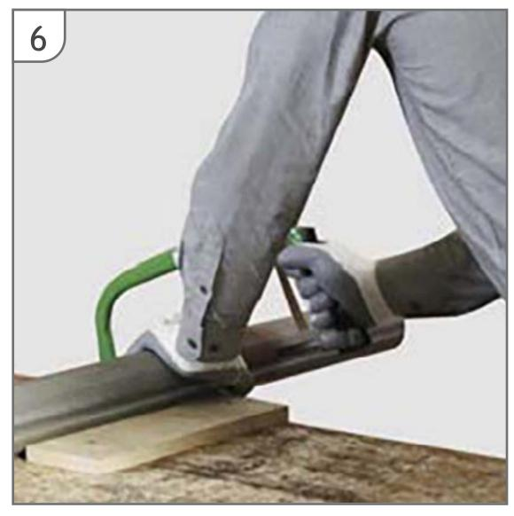
As for the running outlet, when cutting gutter to the required length, always saw from the rolled front edge first.
