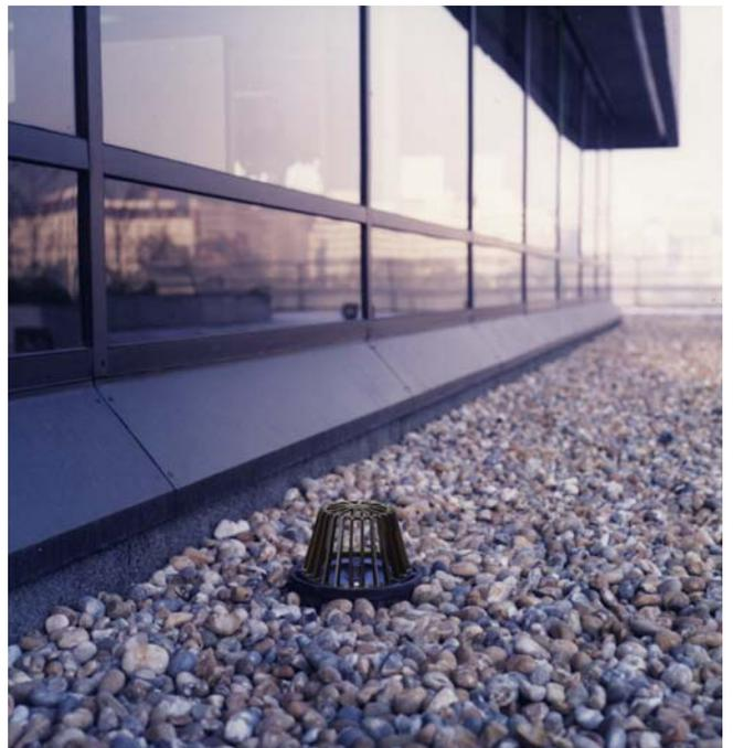
*Variation of a WD Series roof outlet in an inverted roof*
