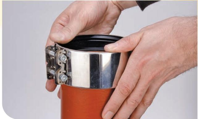
2. Ease-in one side (next to the continuity spur) then push down on the opposite side of the coupling to fully seat, ensuring that the central inner register is abuted against the spigot end.
