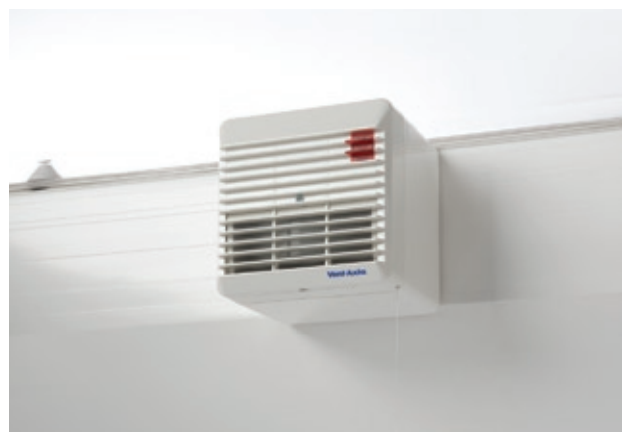
Vent-Axia Solo extract fan 85m 3 /hr (24l/s)
