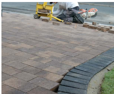
Cutting in of blocks using a block splitter and cutting saw
