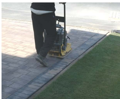
Final 'whacking down' of the paving using a vibration plate
