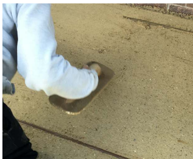
The final laying course of sharp sand being carefully screeded level and smooth
