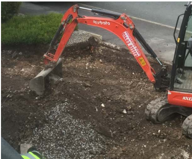
Excavation to the sub-grade level
