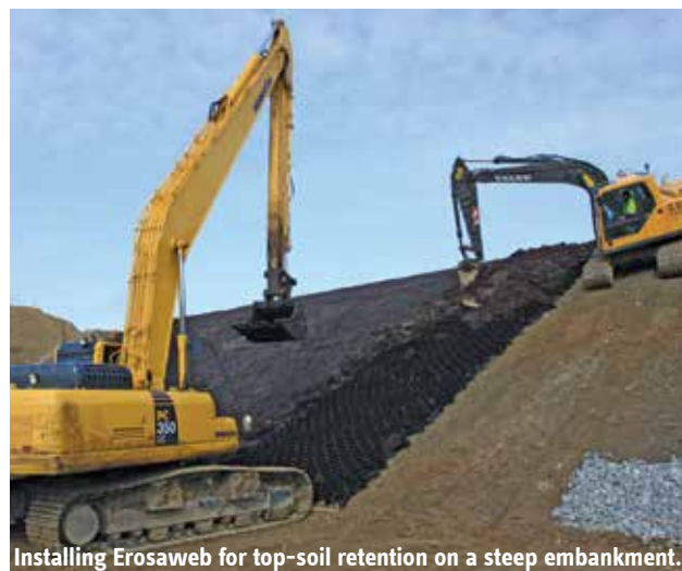
Installing Erosaweb for top-soil retention on a steep embankment.
