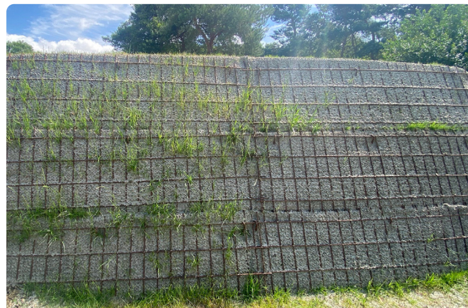
1 Embankment following initial hydroseeding
