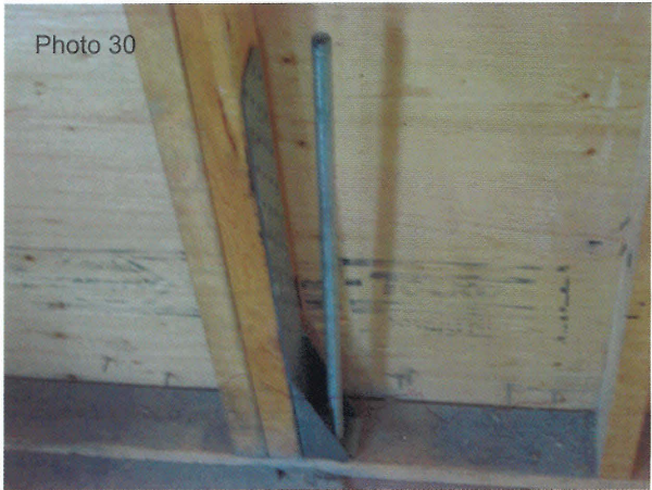
Photo 30 Canada Wood Special connections may be used to transfer forces from floor to floor.
