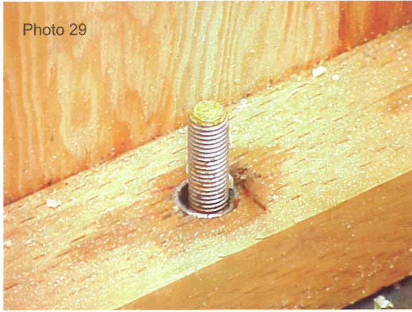
Photo 29 Paul Knight To maximize load transfer, the annular space in the drilled hole is filled with a metal sleeve and grouted.
