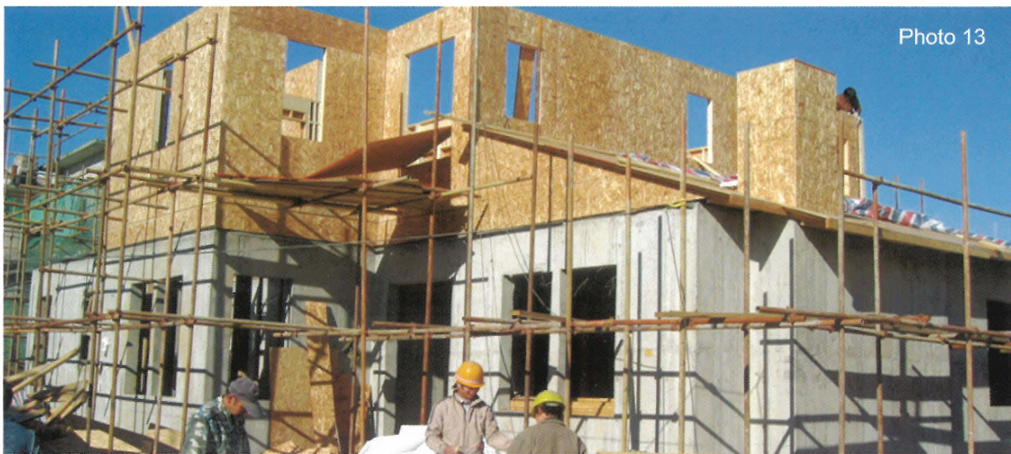
Photo 13 Q-WEB On a smaller scale, wood-framing can be added to a house with a concrete ground floor.
